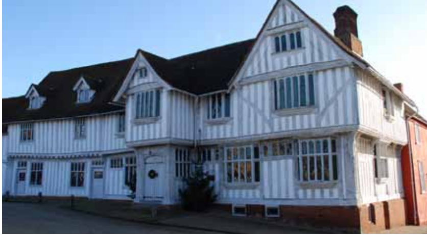
Lavenham Guildhall built towards the end of the economic boom c.1530.
